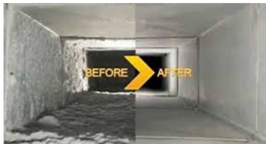
Duct cleaning. (Coil, Duct, Kitchen, Filters)
